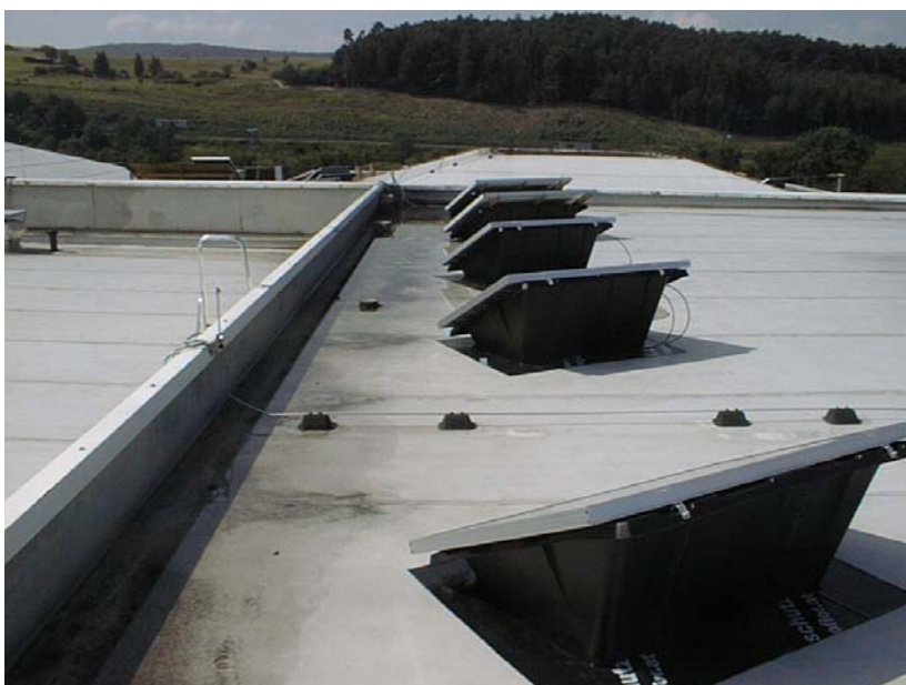
Fig. 2: Example for mounting on ConSole, Ubbink Solar
